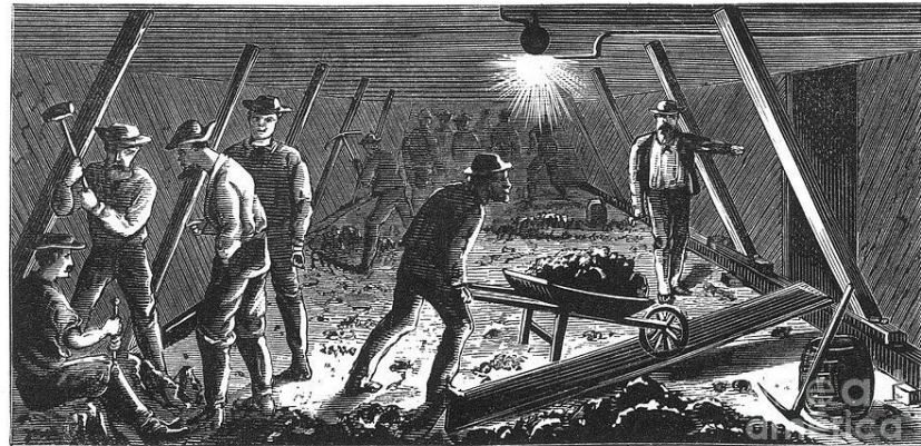
WORKING BENEATH SHOE OR EDGE OF CAISSON.
